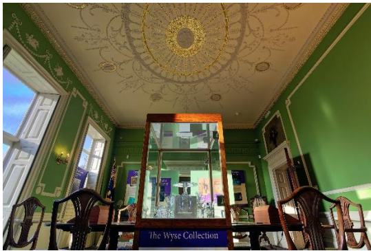
One of the existing plaster ceilings from the 18 th century. © Matt Ling Photography
